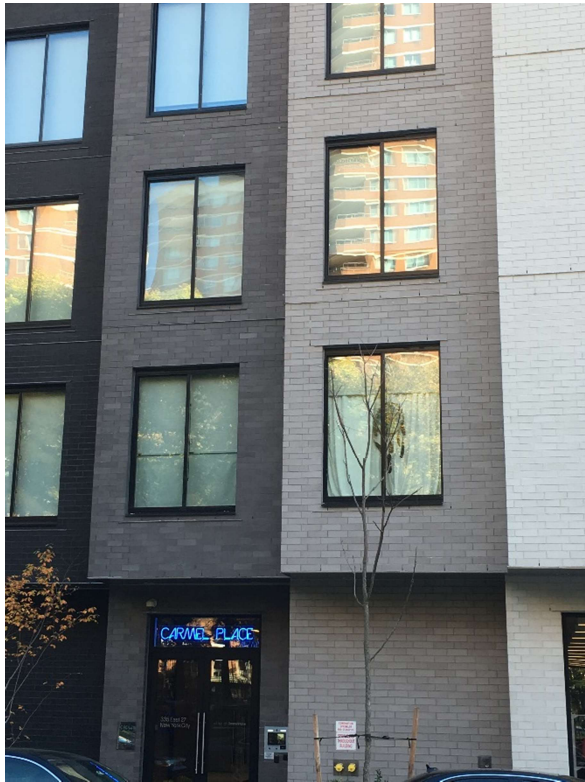
Figure 4: Carmel Place in Manhattan, constructed using modular, prefabricated pieces
